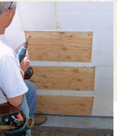
Plywood bandages. After gluing large vertical seams with foam, I reinforce them with plywood scabs screwed to the embedded fastening strips found on both sides of the seams.
