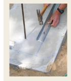
Anchor the first course of ICF blocks by fastening steel track along the chalklines with 1-in. masonry nails spaced about 2 ft. to 3 ft. on center. I set the corners of each course first to eliminate any need to cut, and thereby weaken, this structurally vital part of the foundation.
