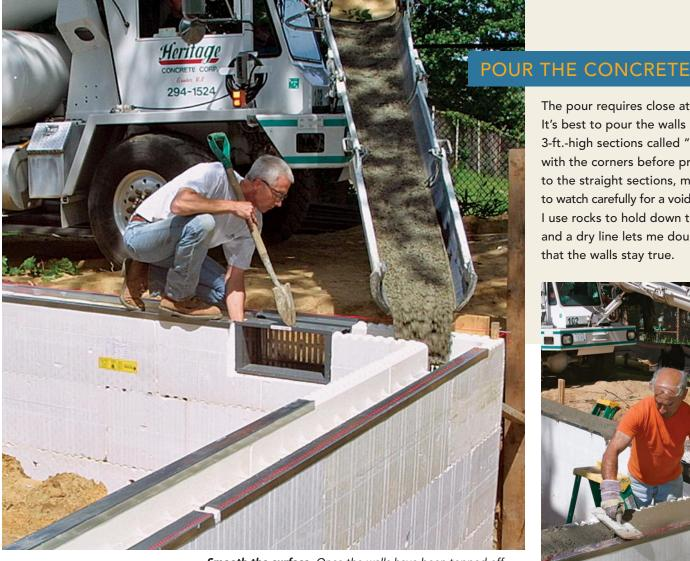
Smooth the surface. Once the walls have been topped off, use steel track as a guide to remove excess concrete and to smooth out the surface before inserting anchor bolts.
