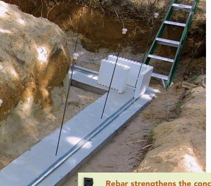
have to compromise their strength by cutting them to fit the rest of the blocks. After I lay the corners, I fill in with straight blocks.
