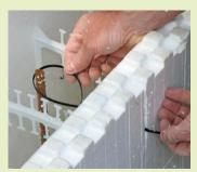
After the first course has been laid, slice the side of one block and loop a zip tie around the vertical rebar that extends from the footing. Pull the tail end of the zip tie through the slot so that it's accessible from outside the form.
