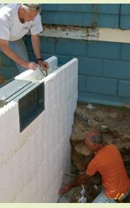
When I drop in another length of vertical rebar from above, it is carefully threaded into the looped zip tie, which then is pulled tight with a pair of pliers to tie the rebar together.
