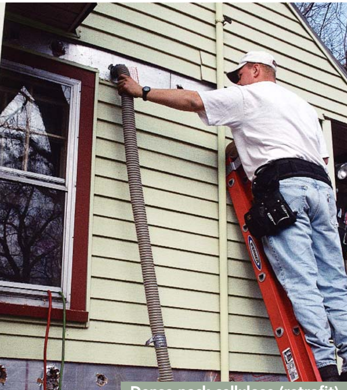
Dense-pack cellulose (retrofit)
