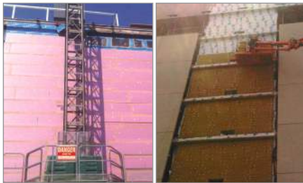
Exterior walls - Insulation to concrete
