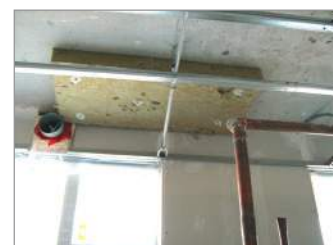
Ceiling acoustical insulation
