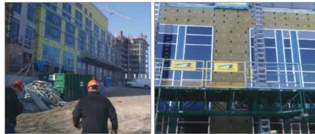
Exterior walls - Insulation to steel stud
