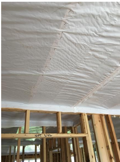
Poly on 2 nd floor ceiling
