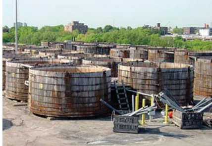
Tank staves have vertical grain. Storage tanks, such as these Bick's pickle tanks outside Toronto, required clear, straight grain to limit movement and prevent leaks.
