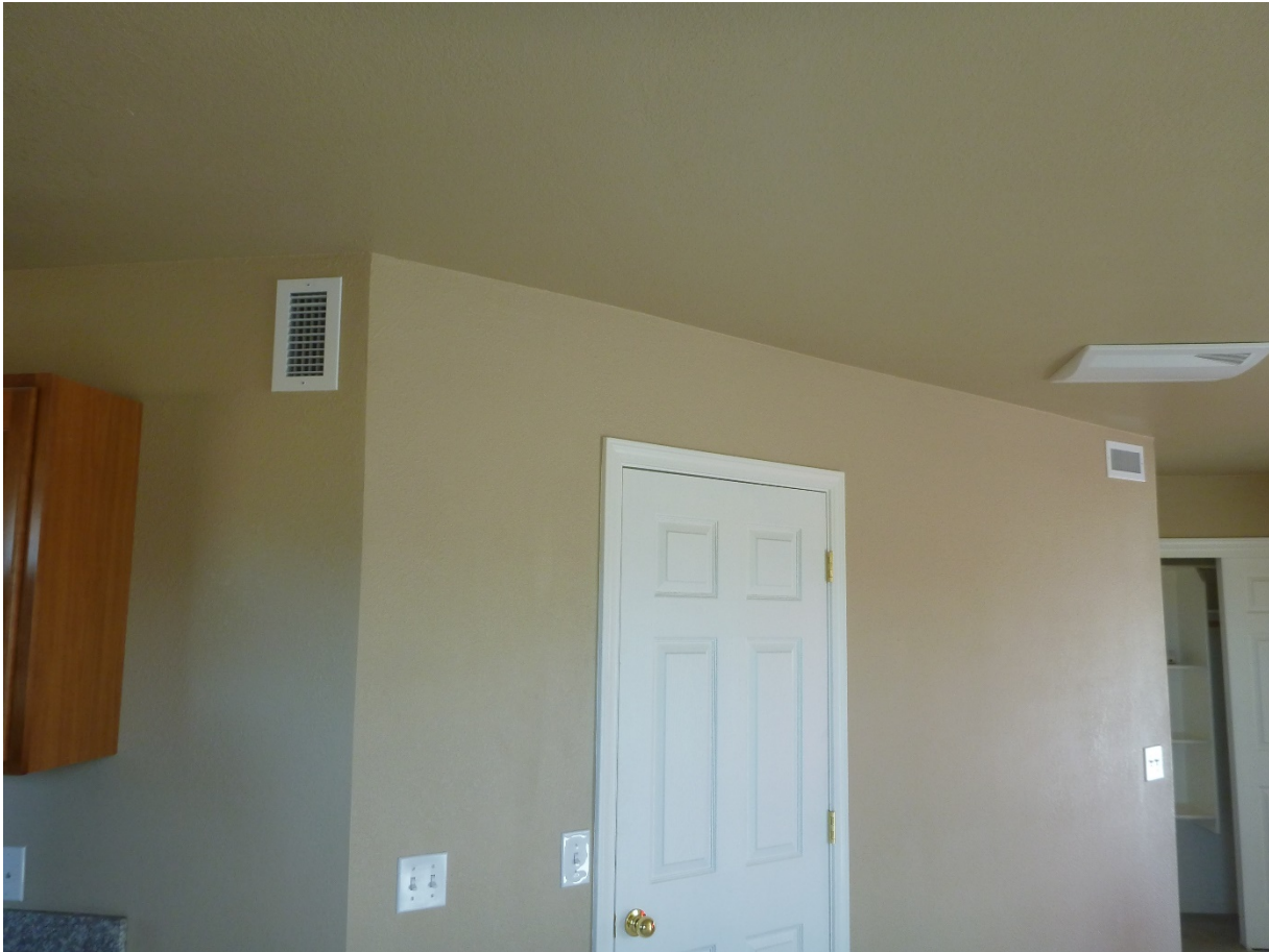
Figure A3.39 Double-deflection Supply Grilles (Chitwood Energy Management)
