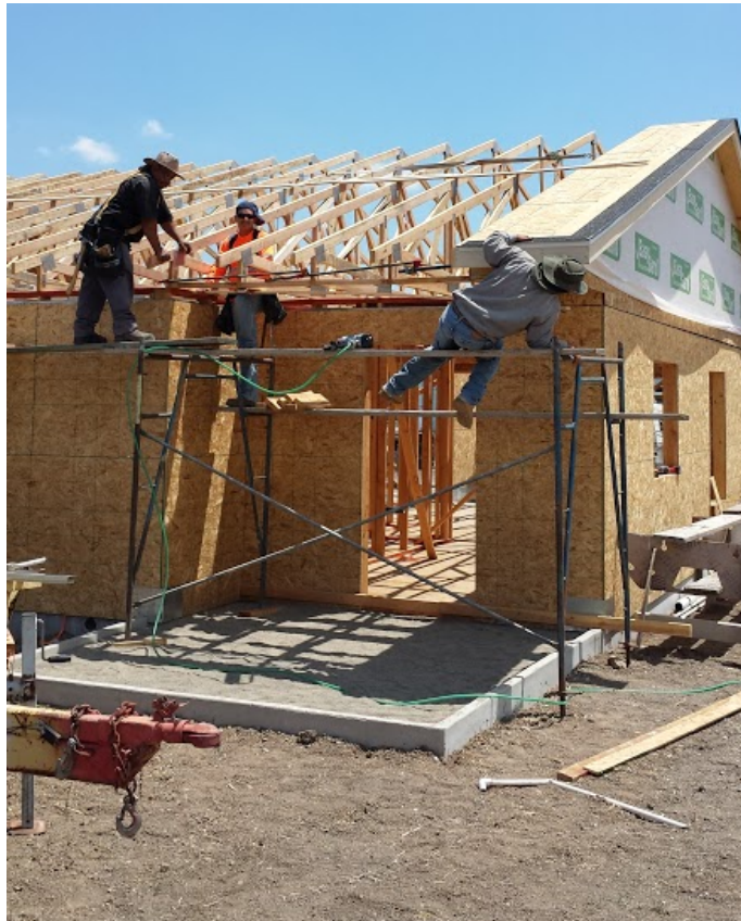
Figure A3.21 Gable End Truss in Place (Chitwood Energy Management)
