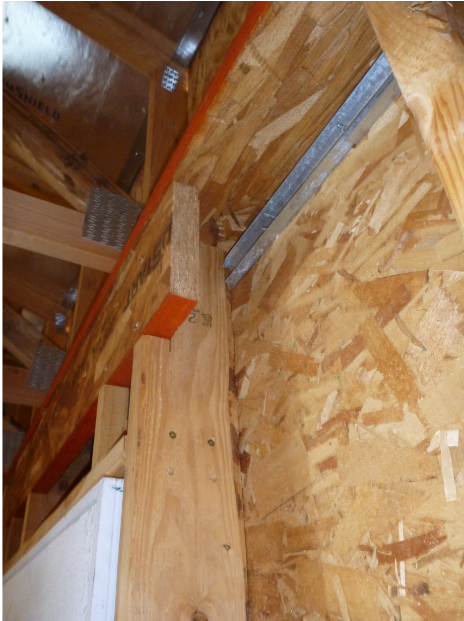
Figure A3.17 Engineered Headers. (Chitwood Energy Management)
