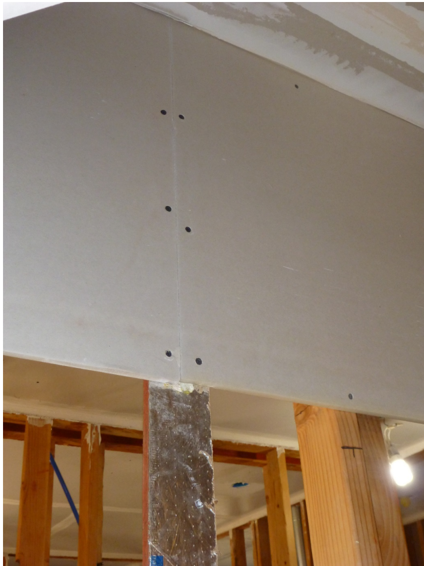
Figure A3.18 Drywall Splicing (Chitwood Energy Management)
