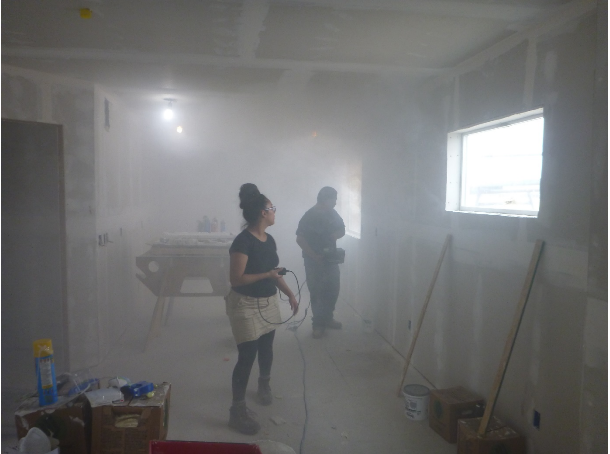
Figure A3.29 Smoke Testing (Chitwood Energy Management)
