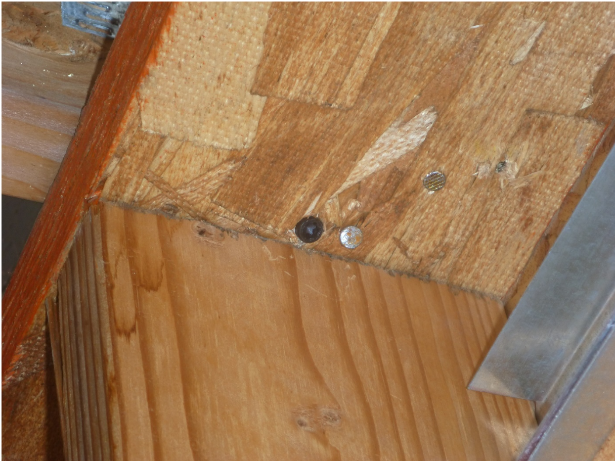
Figure A3.23 Truss Hold-down Screws (Chitwood Energy Management)
