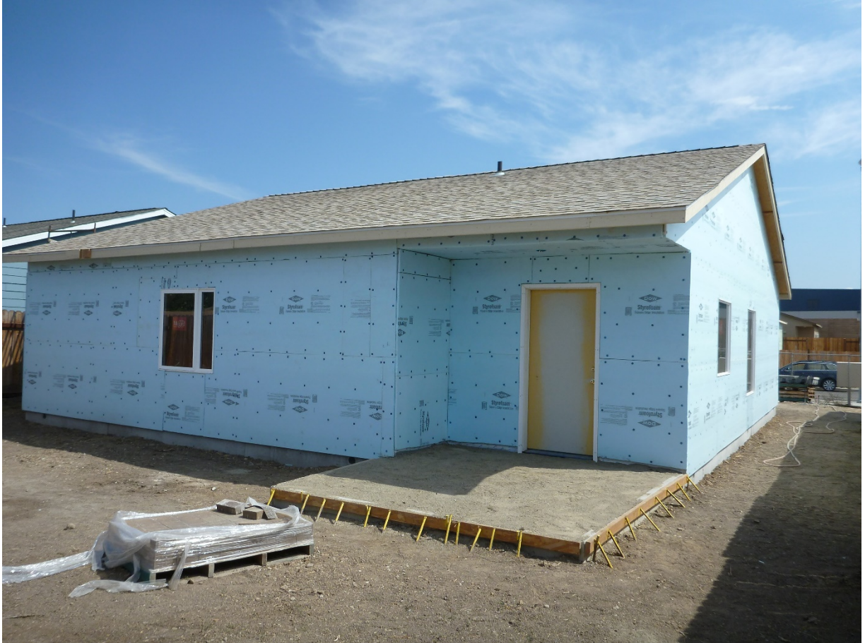
Figure A3.26 Cantilevered Porch (Chitwood Energy Management)
