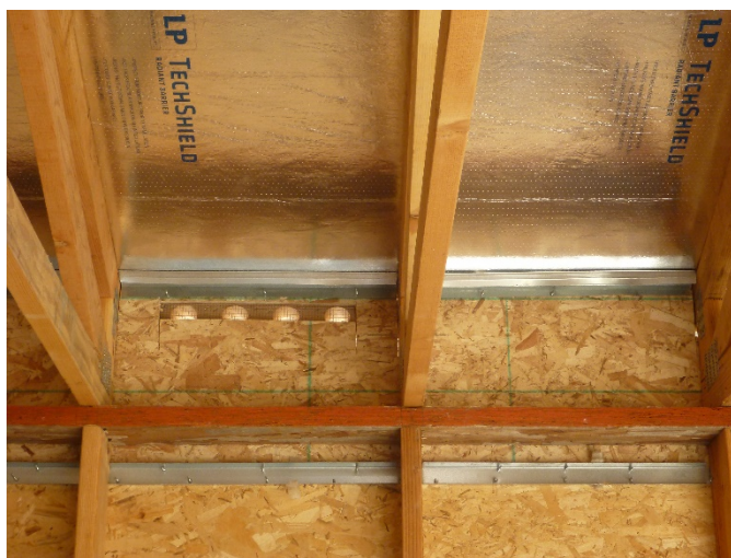
Figure 11. Truss Assembly (Chitwood Energy Management)
