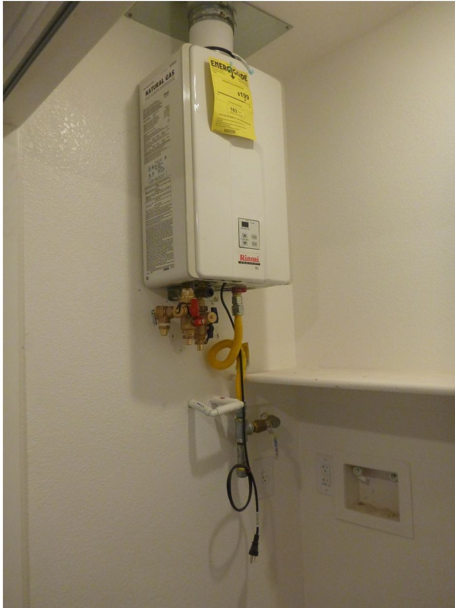
Figure A3.40 Tankless Water Heater (Chitwood Energy Management)
