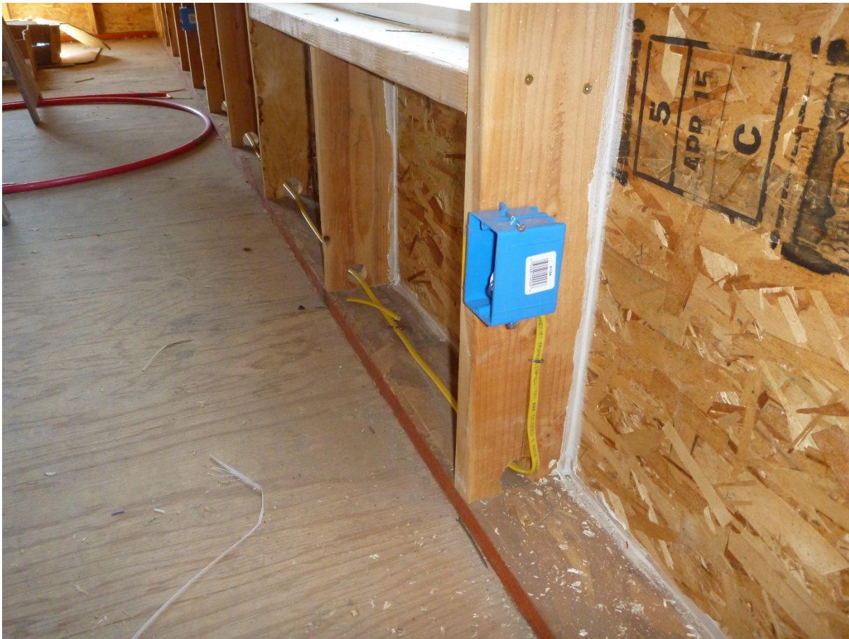
Figure A3.27 Studs Pre-drilled for Wiring (Chitwood Energy Management)
