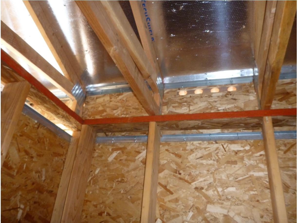
Figure A3.30 Raised-heel Trusses (Chitwood Energy Management)
