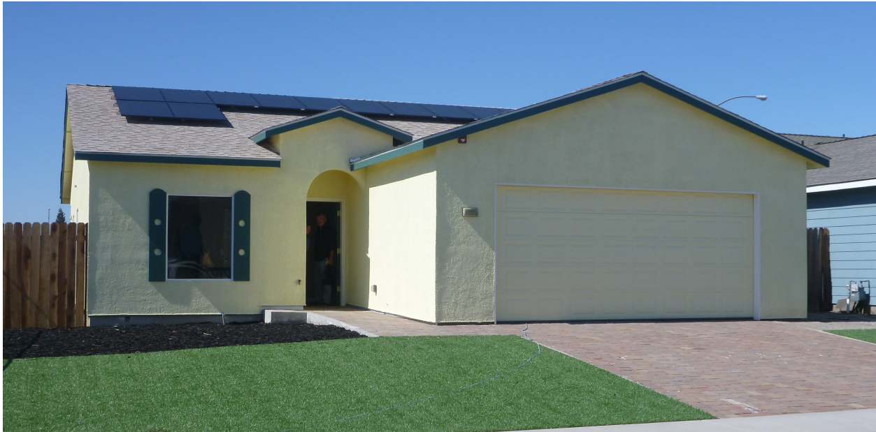
Figure 1. Completed Demonstration Home (Chitwood Energy Management)
