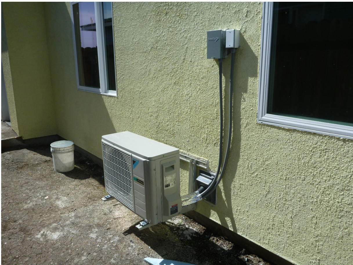
Figure A3.36 Mini-split Heat Pump (Chitwood Energy Management)
