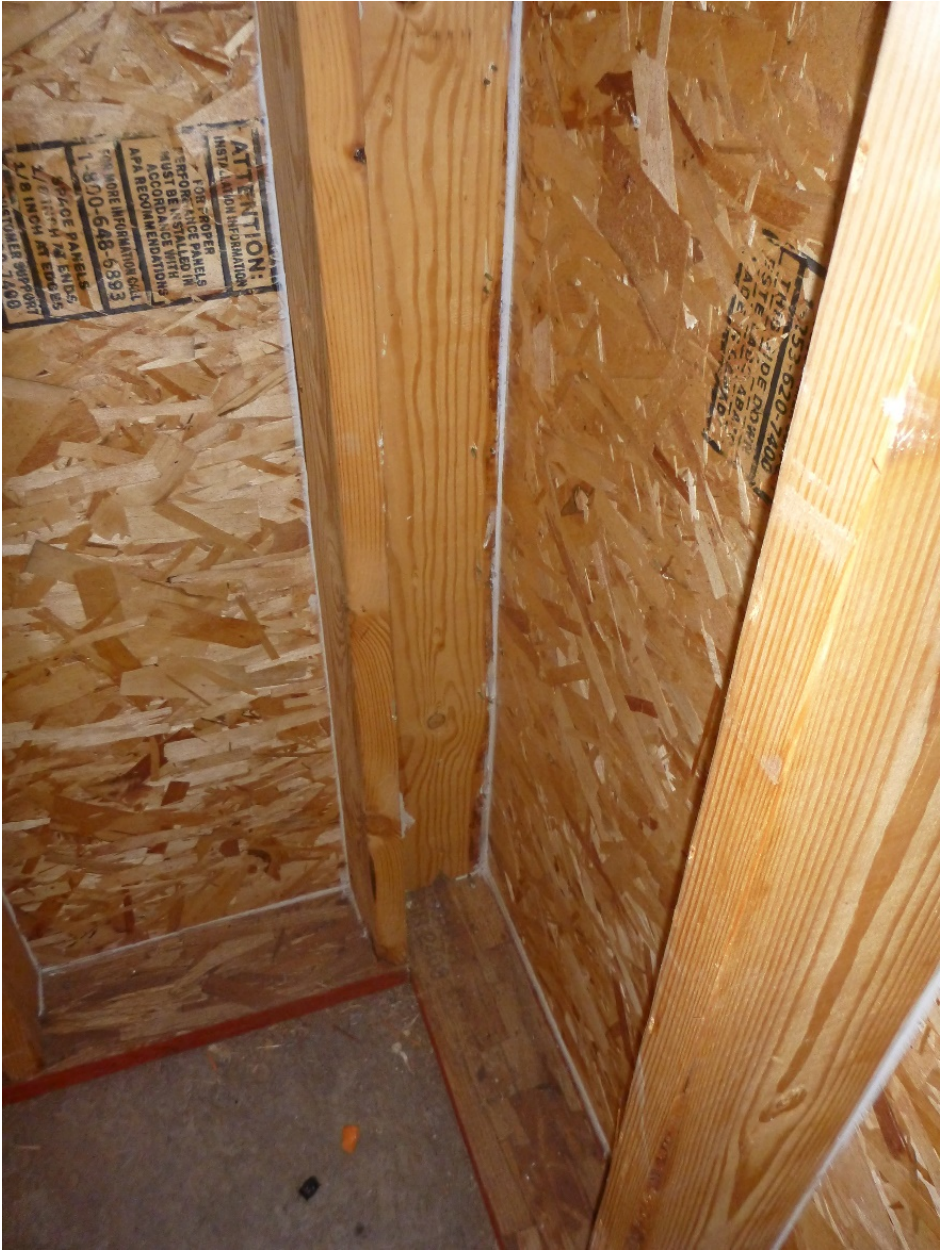
Figure A3.12 Two-stud Corners (Chitwood Energy Management)
