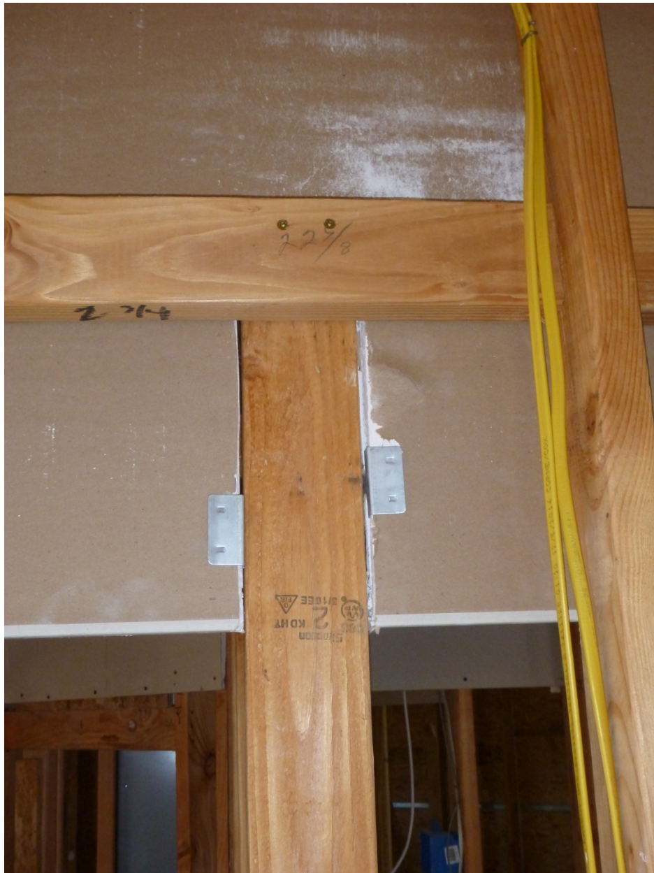
Figure A3.16 Drywall Clips (Chitwood Energy Management)
