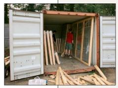
A white-glove inspection. After cracking open the locked shipping container, the window reps remove all of the bracing and inspect the windows and doors for damage. Upon approval, the units are then signed over to the builder.
