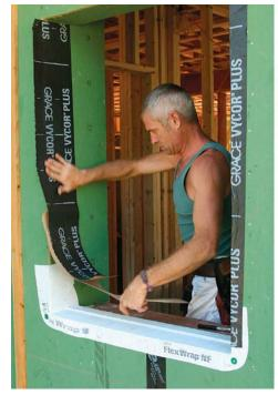
Seal the vertical seams. The sides of the rough opening, where the exterior sheathing meets the boxed window-frame assembly, are protected with lengths of Grace Vycor flashing, which lap over the sill flashing.
