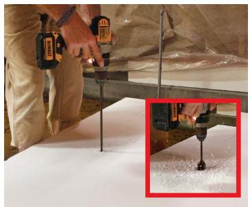
**Drill from both sides.** When you need to drill holes for pipes and other penetrations in the thick foam, a standard spade bit or hole saw won't be long enough. Instead, use a long bellhanger-style drill bit to bore a pilot hole all the way through the foam. Then, using a standard spade bit, widen the pilot hole from both sides of the panel. For holes of a larger diameter, skip the drill bits and go right for the reciprocating saw.
