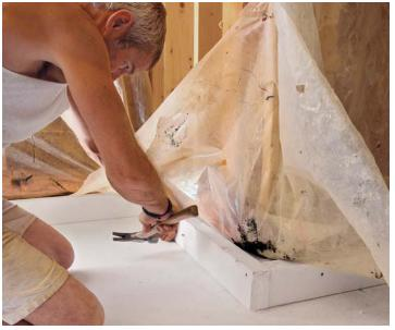
**Tack on the edge.** The innermost pieces of perimeter foam come last and act as the screed level for the concrete slab. After applying a bead of spray foam to the outer perimeter foam, a worker tacks the inside pieces to that first layer of foam with nails every few feet to keep them from shifting until the spray foam sets up.
